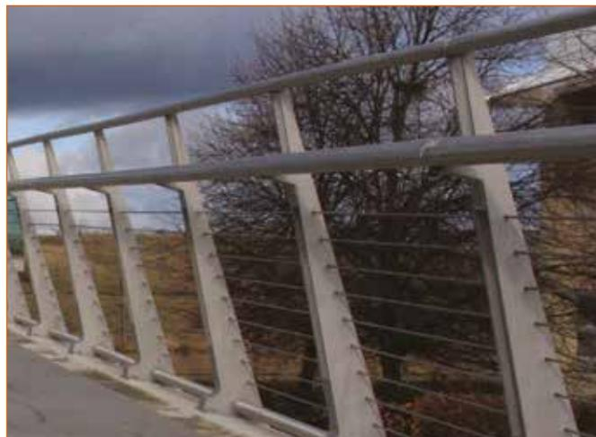
**Inwardly inclined support posts and offset horizontal rails improve safety**
