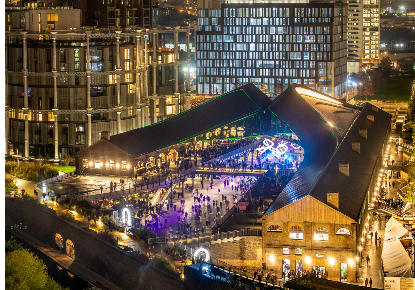
LABC Building Excellence award winner Coal Drops Yard, Kings Cross
